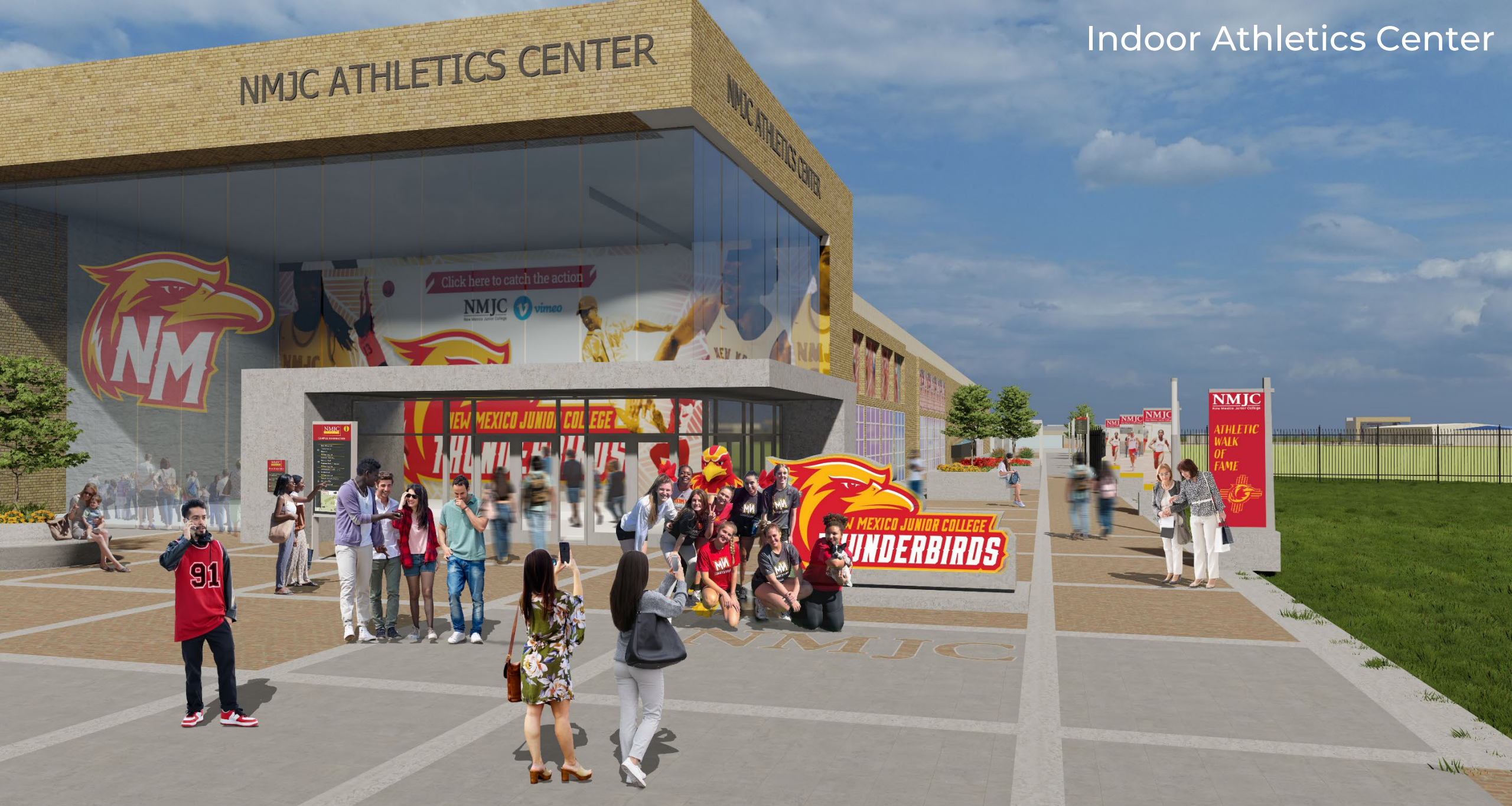
A new indoor Athletics Center anchors the larger Athletics District. It is intended to host regional and national track and field events.
