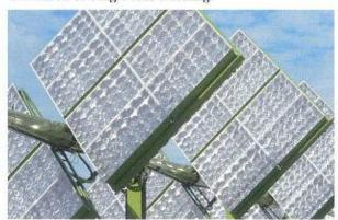
The Green Volts CPV System is currently being used for utility scale installations in excess of 2mW. One benefit to using CPV is that the cells do not loose efficiency due to high temperatures. Traditional PV panels see a decreased drop in efficiency when temperatures rise. The Green Volts CPV remains efficient regardless of outside ambient temperature. The Green Volts CPV
